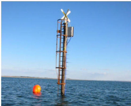
Figure 3, example of marking: Yellow cross on mooring pile and orange buoy at mooring line
