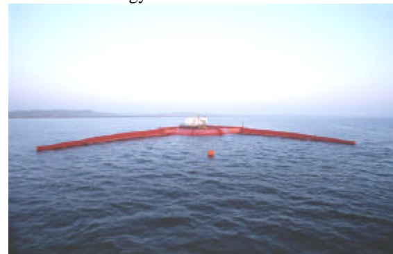
Figure 2, photo from the first deployment site of Wave Dragon with reflectors, platform and container
