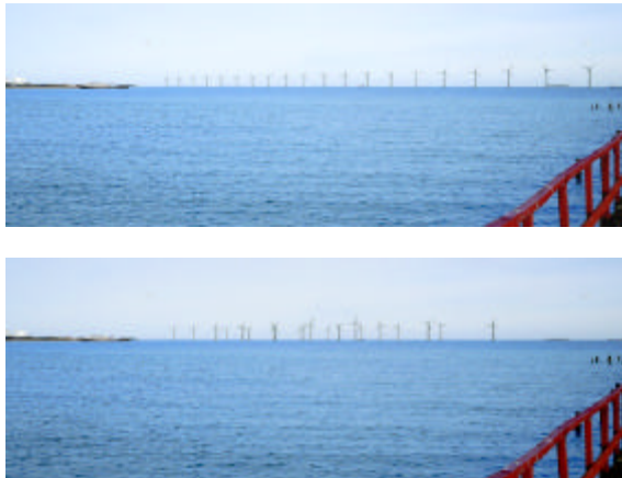
Figure 2 The Middelgrunden “the three rows” and “the curved line” from the beach at Kastrup [11]
